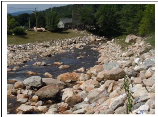
Dam Removal and Plantings on North Branch of the Hoosic River
